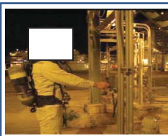
AN Field operator wore SCBA and performed isolation valve at Plant.
